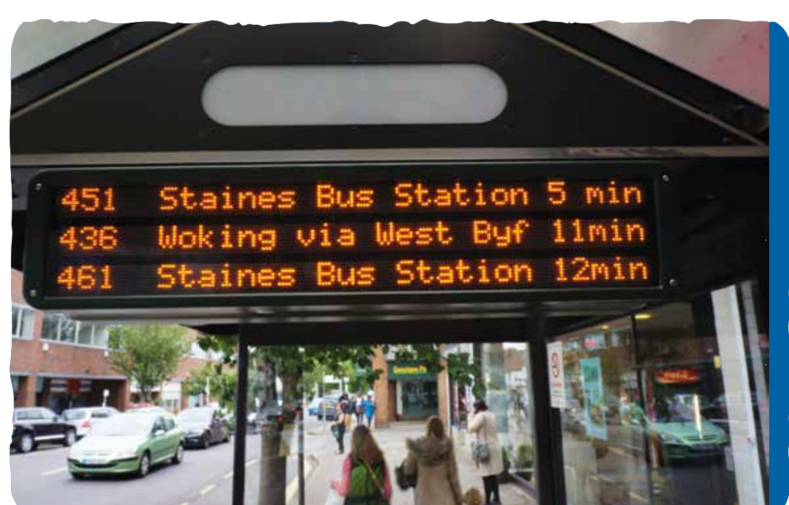
Real time passenger info will be available at bigger bus stops along routes
